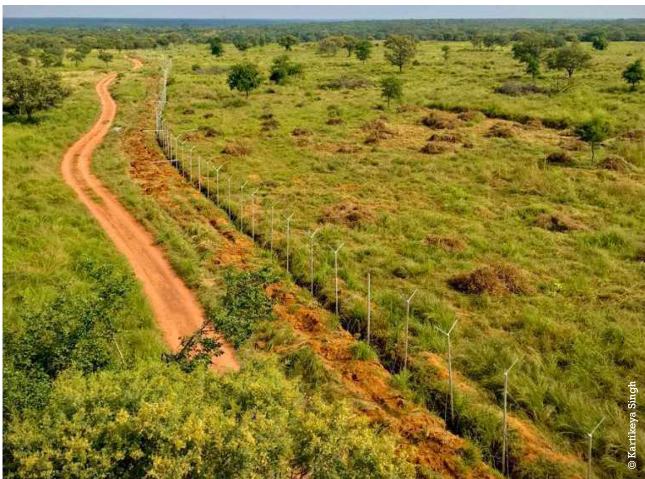
Image 7. Predator proof fenced enclosure under construction for soft release of cheetahs in Kuno National Park.
